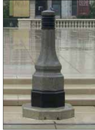
Standardized utility hookups can be disguised in bollards, reducing the need for temporary facilities. Shown are utility hookups in Ottawa (left and center) and a utility bollard in Chicago's Millennium Park (right).
